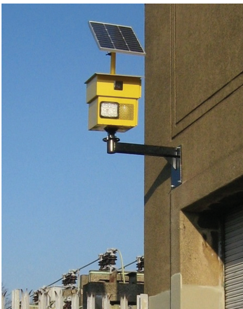
The cameras and AEGIS UFLED White Light Illuminators are housed in imposing yellow boxes.
